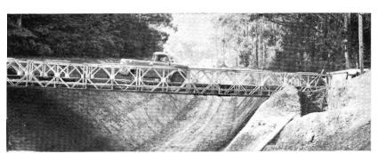
THIS army type "Bailey" bridge provides a temporary roadway at McNicol Road, Tecoma. A new concrete and steel structure will be built there.
