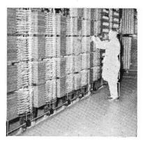
PORTION of the intricate switching equipment in the 2,500 line automatic telephone exchange in the V.R. Head Offlice.
