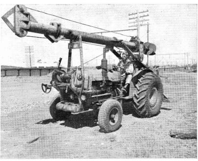
(Above) THIS machine is a combined earth borer and pole erector. As it here backs into position at St. Albans, the boring member is astride the petrol-driven vehicle. The driver mechanically tilts the borer—which has an interchangeable, rotating auger—to make the hole. After the machine hoists the pole, fixing is completed by manpower.
