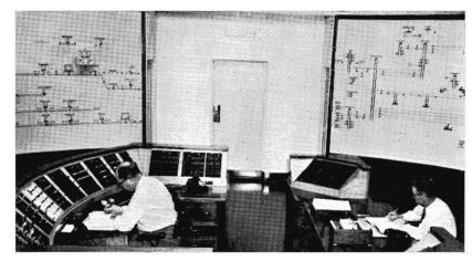
POWER Operations Room at Batman Avenue, Melbourne. On the walls are indicated the operational points in the suburban electrified area. The Power Operation Engineer (left) controls the distribution of electric power throughout the suburban system. A clerk (right) keeps a complete daily record of operations carried out in the room.
